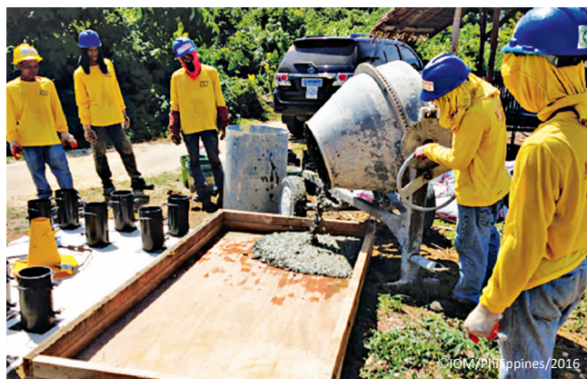
Random materials testing on site
